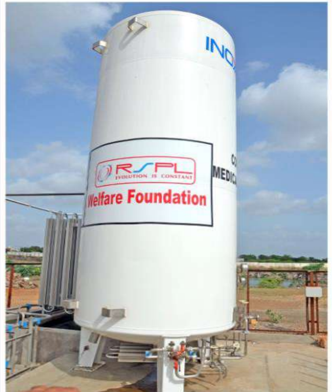
Installed 9KL Capacity Oxygen Tank alongwith Vaporizer system at Khambhalia General Hospital to combat Covid-19 pandemic
