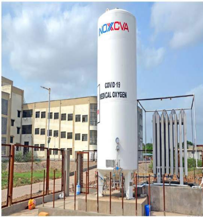
Installed 9KL Capacity Oxygen Tank alongwith Vaporizer system at Khambhalia General Hospital to combat Covid-19 pandemic
